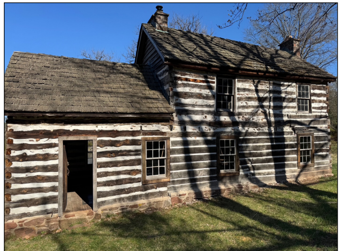
The back side of the Willard Log Cabin
