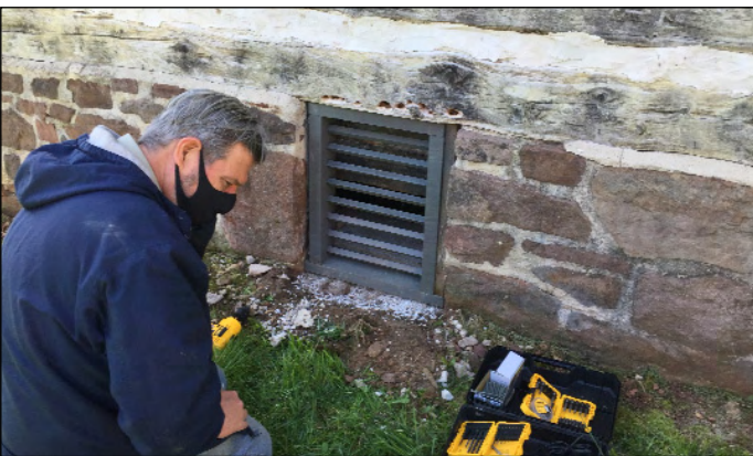
Rebuilt Root Cellar Vent
