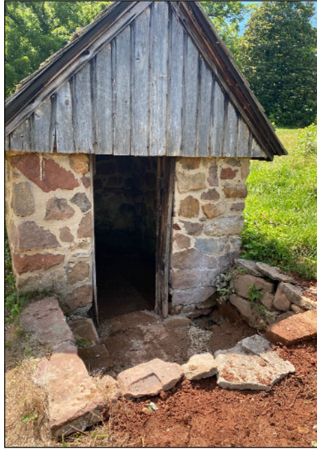
Repaired stone work
