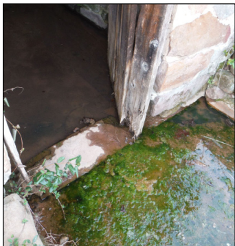
Spring house - dammed-up water flow
